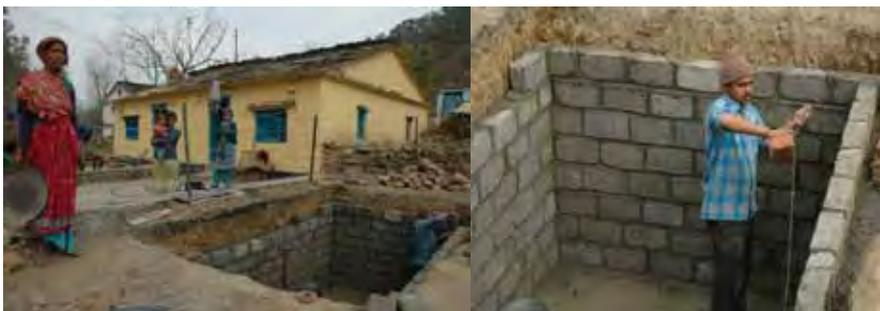
Random rubble concrete blocks could be made locally and used for construction of storage tanks
